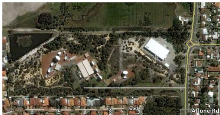
Figure 4: Lockridge Earth Station
